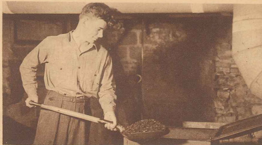
Eliminating winter drudgery —that's the job done by this automatic stoker powered by a ¼ HP electric motor. Once a day during the cold months Dick Woody loads the stoker with inexpensive pea-size coal, the motor does the rest keeping a clean, even fire burning in their central heating furnace.
